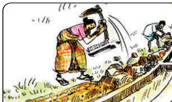
Digging trench and keeping soil downstream side
