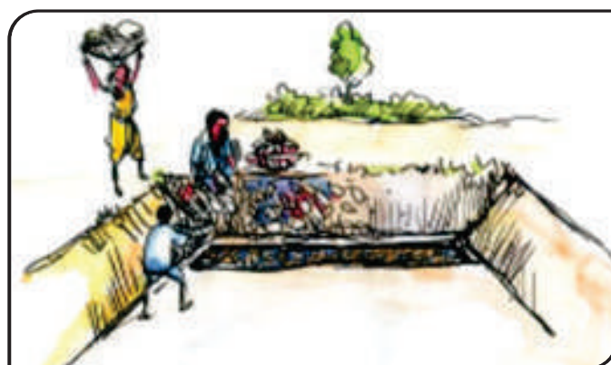
Constructing stone revitment
